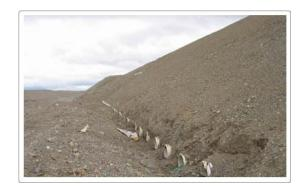
In some places, the engineers buried ventilation pipes in the ground. The pipes simply allow the cold air to circulate underneath the rail-bed. In other spots, though, a pipe called a thermosiphon was sunk 5 meters (15 feet) into the ground and filled at the bottom with ammonia A monitoring system has been established to check the temperature change along the railroad.
