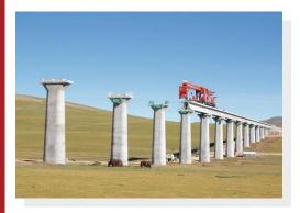
Permafrost areas were avoided as possible, by building bridges instead of railroad. Building a bridge over the permafrost, though expensive, has the least impact on the area. The 11.7km Qingshuihe Bridge is the world-longest bridge built on permafrost.
